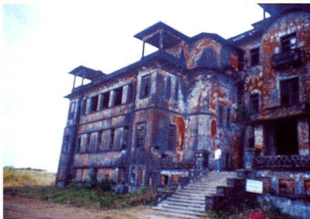
Nekdanji hotel in casino Bokor Hill.
